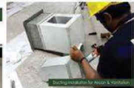
Ducting Installation for Aircon & Ventilation
